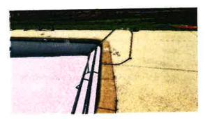
The pool plaster appeared to be in condition expected given the age of the plaster. Staining, rough spots and minor areas of delamination were observed.
