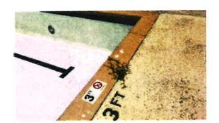
No Diving and depth markers are inconsistent, faded and not easily visible. Joint between deck and coping should be cleaned and caulked.
