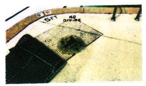
The pool deck showed numerous areas where the deck topping was worn and the underlying concrete deck was visible. Although the majority appears serviceable at this time, there are cosmetic concerns and some cracks and offsets should be addressed. Cracks left unrepaired can contribute to further deck issues down the road.
