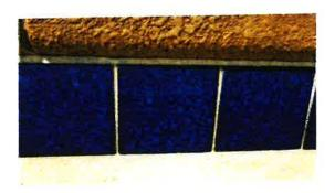
Waterline tile was sound, and no evidence of delamination were observed. The marker and racing lane tile in the pool all appeared to be in fair condition. Grout joints at marker and step tile were missing grout in many places.
