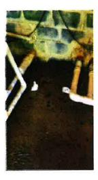
The pool equipment room was not dry, a properly functioning floor drain system was not observed. The overall condition did not appear to meet the code requirements. The filter plumbing had been replaced at some point. The new plumbing is of insufficient sizing does not meet code. Appears serviceable but the concerns above should be addressed and corrected. The pool pump and recirculation system were not operated nor tested.
