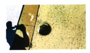
It appears that the original pool coping was removed at some point and replaced with a poured in place coping. The current coping and textured topping is in poor condition showing cracks, spalling concrete, and delaminated topping. There is no expansion joint between the deck and coping.
