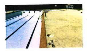
The pool structure appears to be sound and there was no visible cracking or other indication of sub-sub surface shell/concrete issues.
