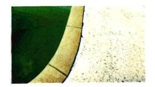
Several areas of the deck have settled and are not flush with the pool coping. The joint between the deck and pool coping shows cracking, spalling, and chipping. Appears serviceable but should be investigated and repaired if needed.
