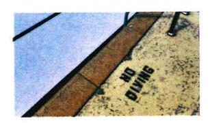
Chipping and cracking at deck to coping transitions should be repaired.
