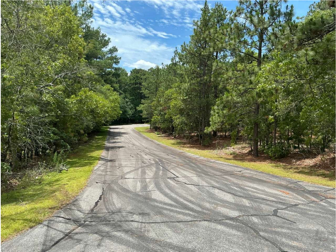
Asphalt Paving & Repairs
