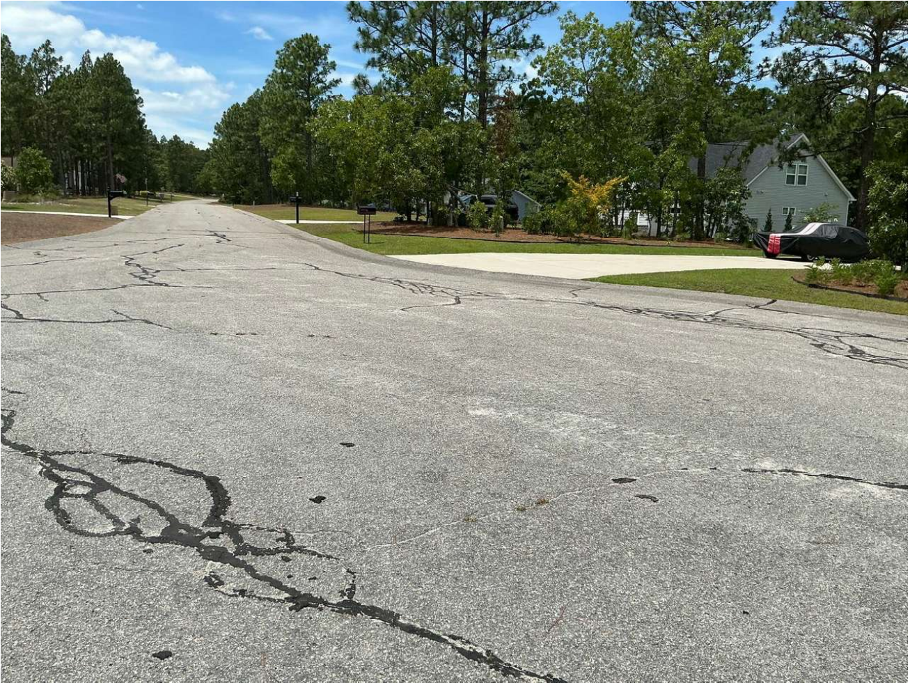
Asphalt Paving & Repairs
