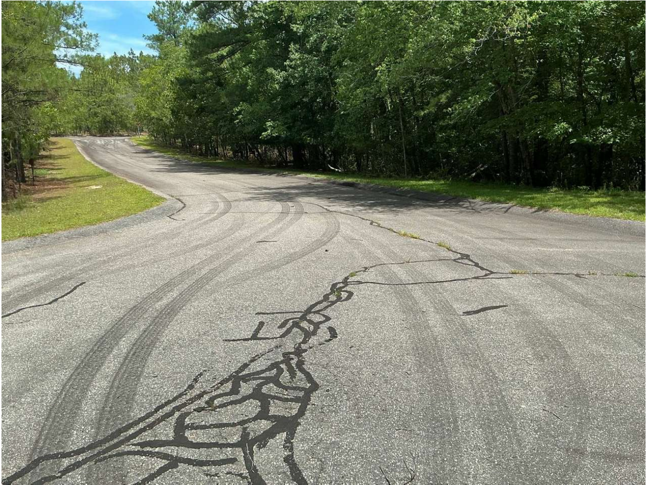
Asphalt Paving & Repairs
