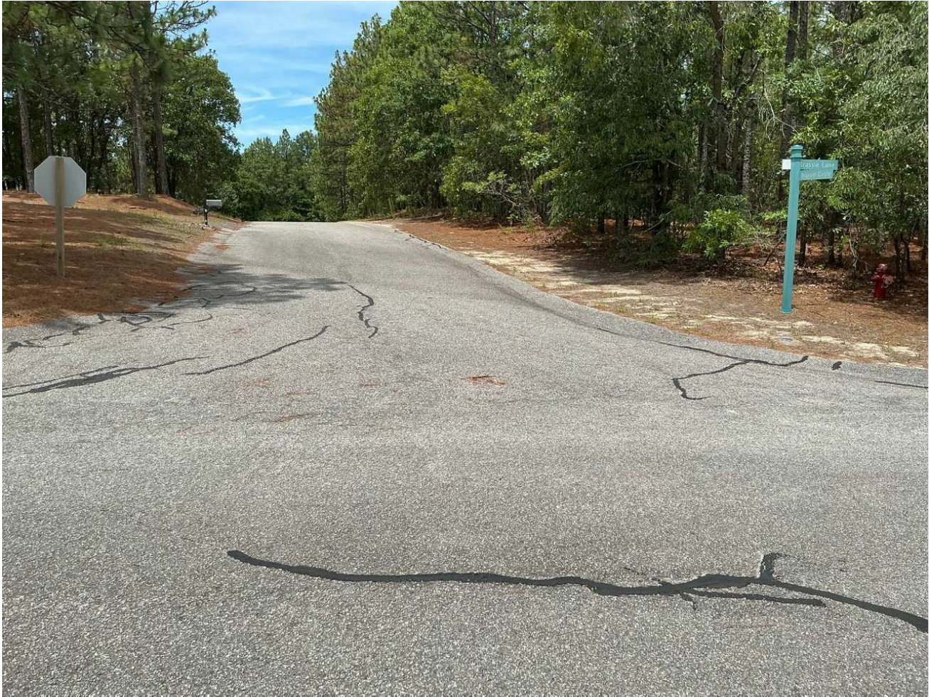
Asphalt Paving & Repairs
