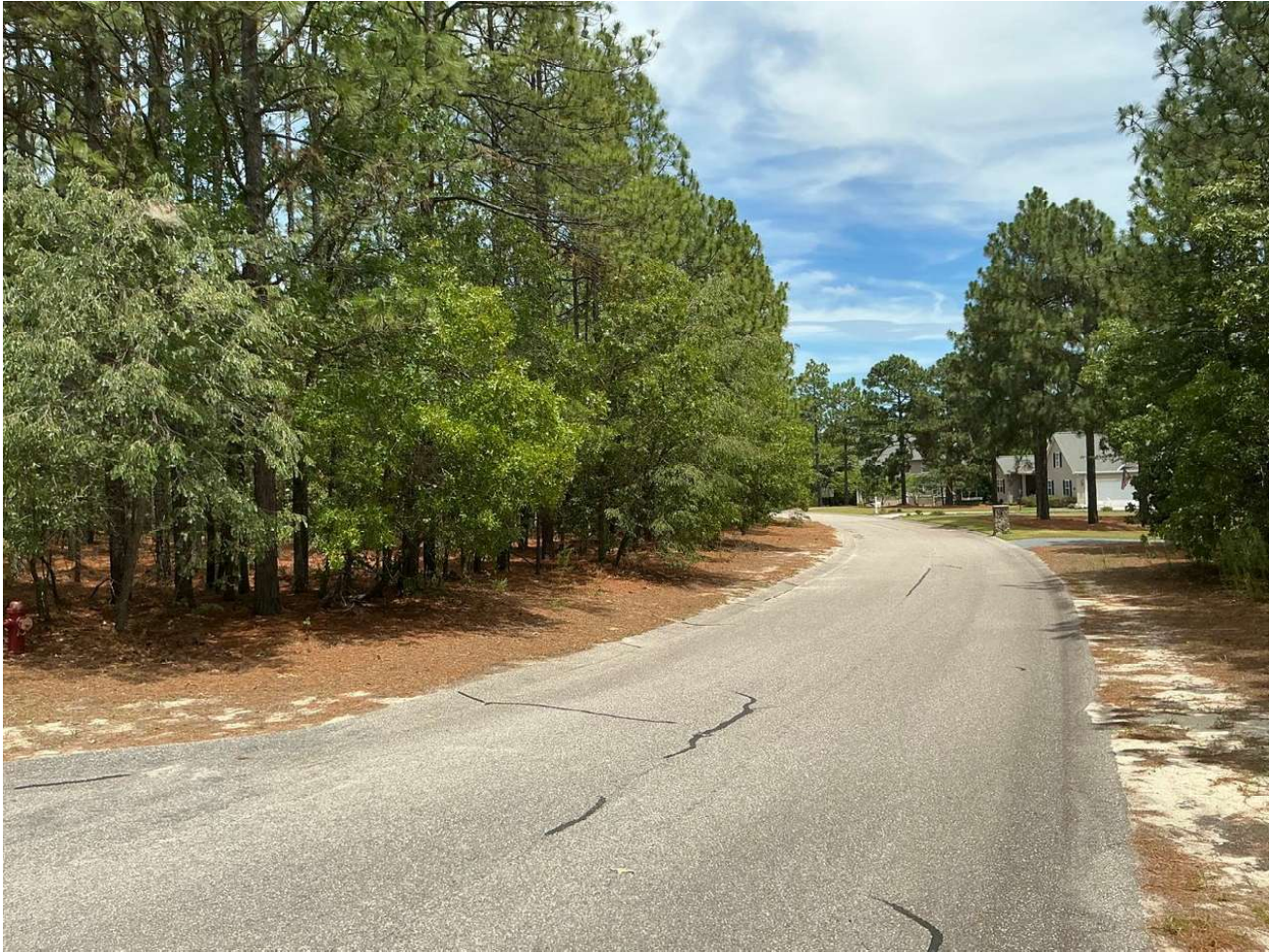
Asphalt Paving & Repairs
