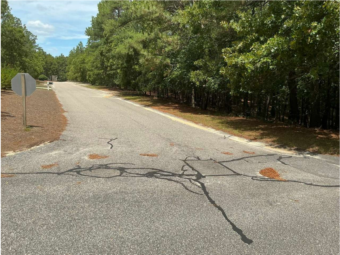
Asphalt Paving & Repairs
