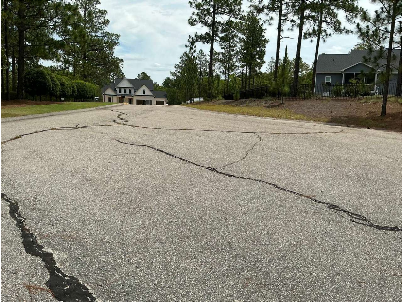
Asphalt Paving & Repairs
