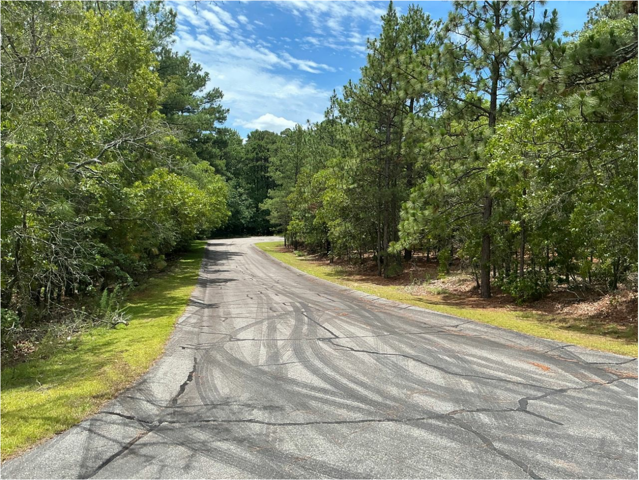
Asphalt Paving & Repairs
