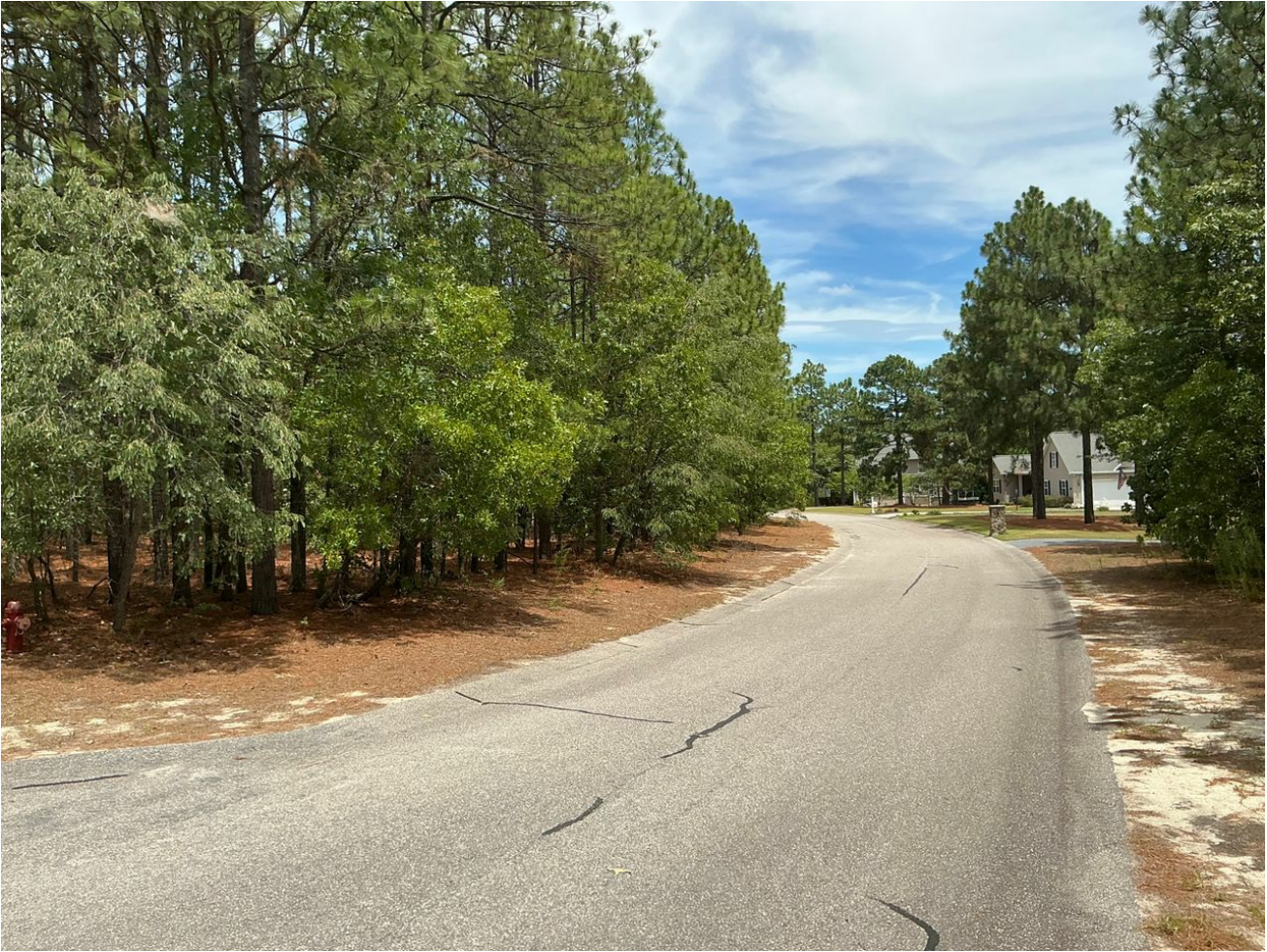
Asphalt Paving & Repairs
