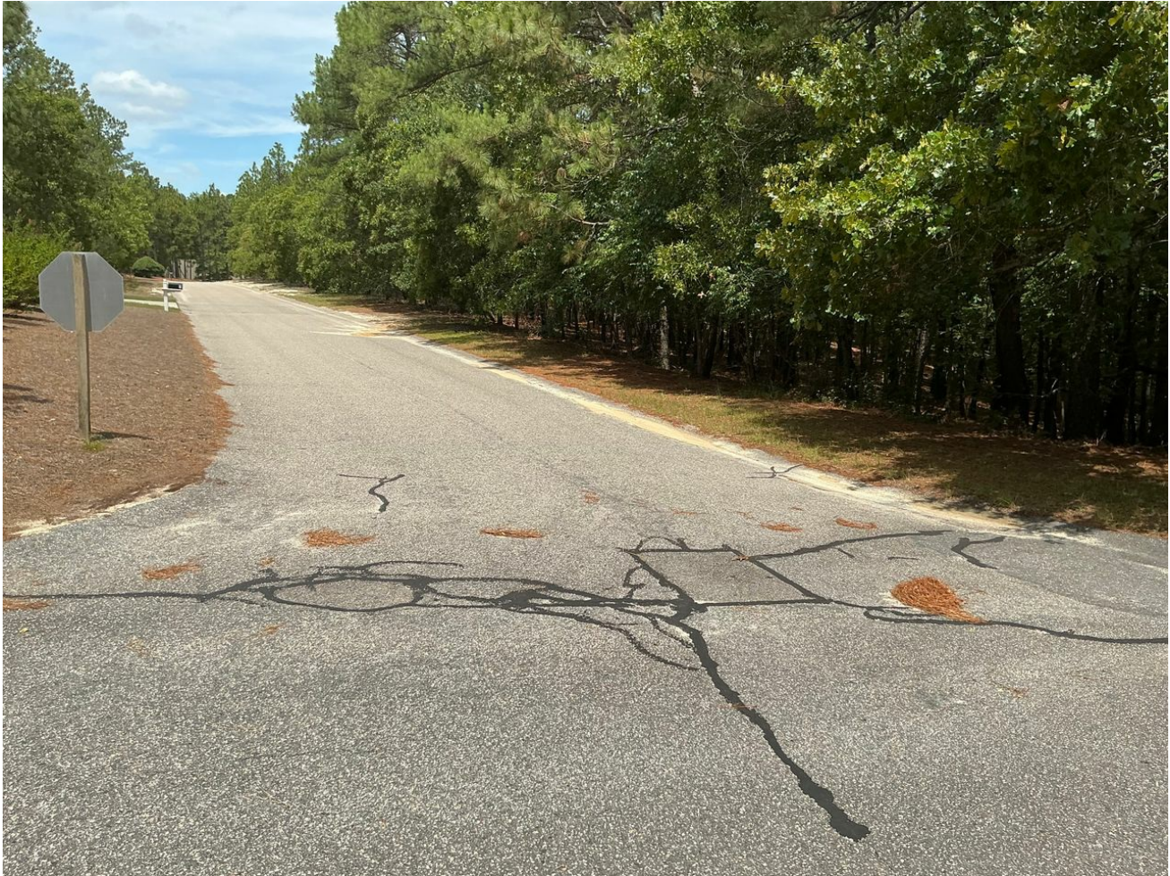
Asphalt Paving & Repairs
