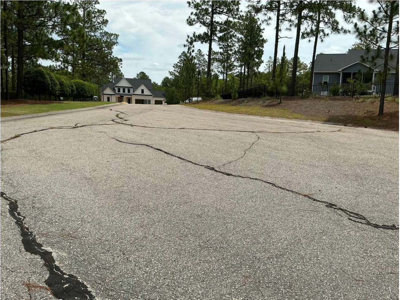
Asphalt Paving & Repairs
