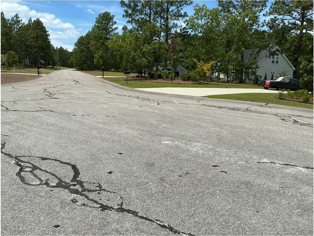
Asphalt Paving & Repairs
