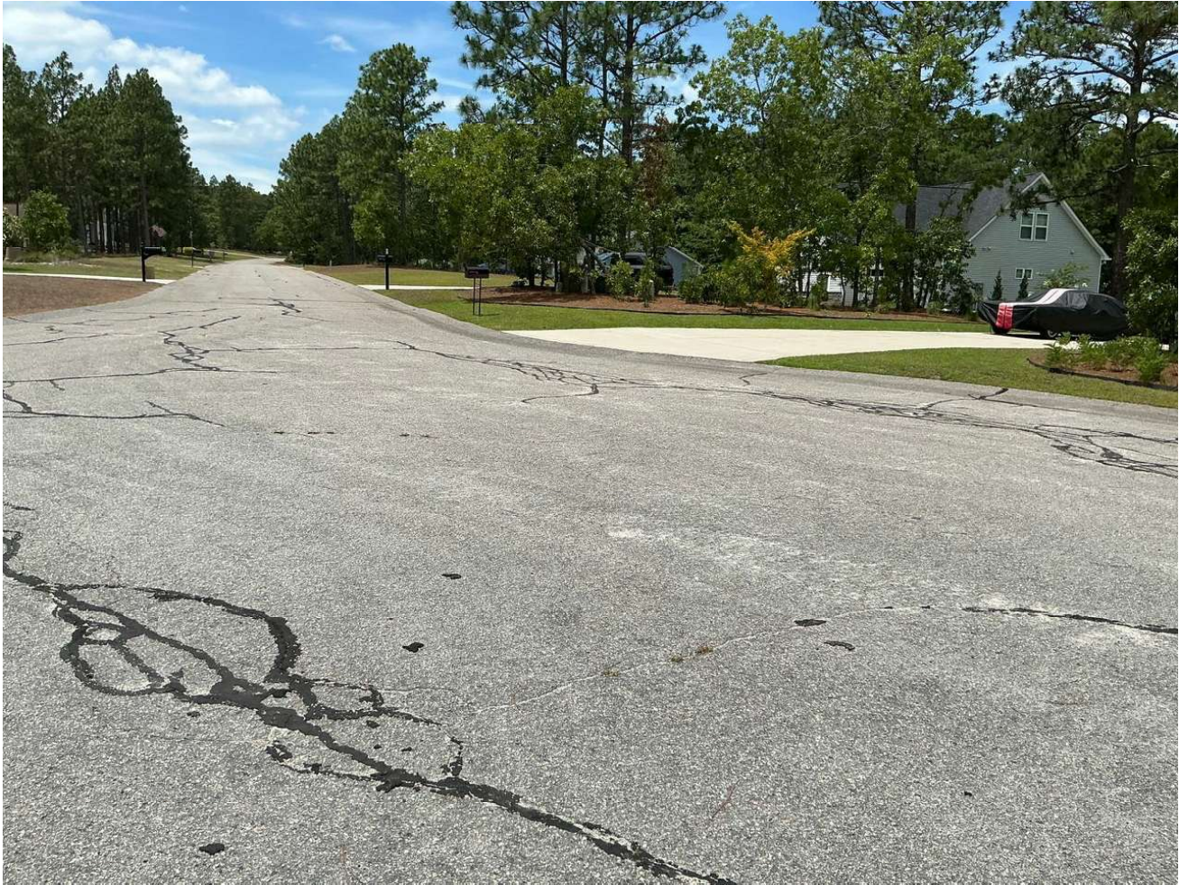
Asphalt Paving & Repairs
