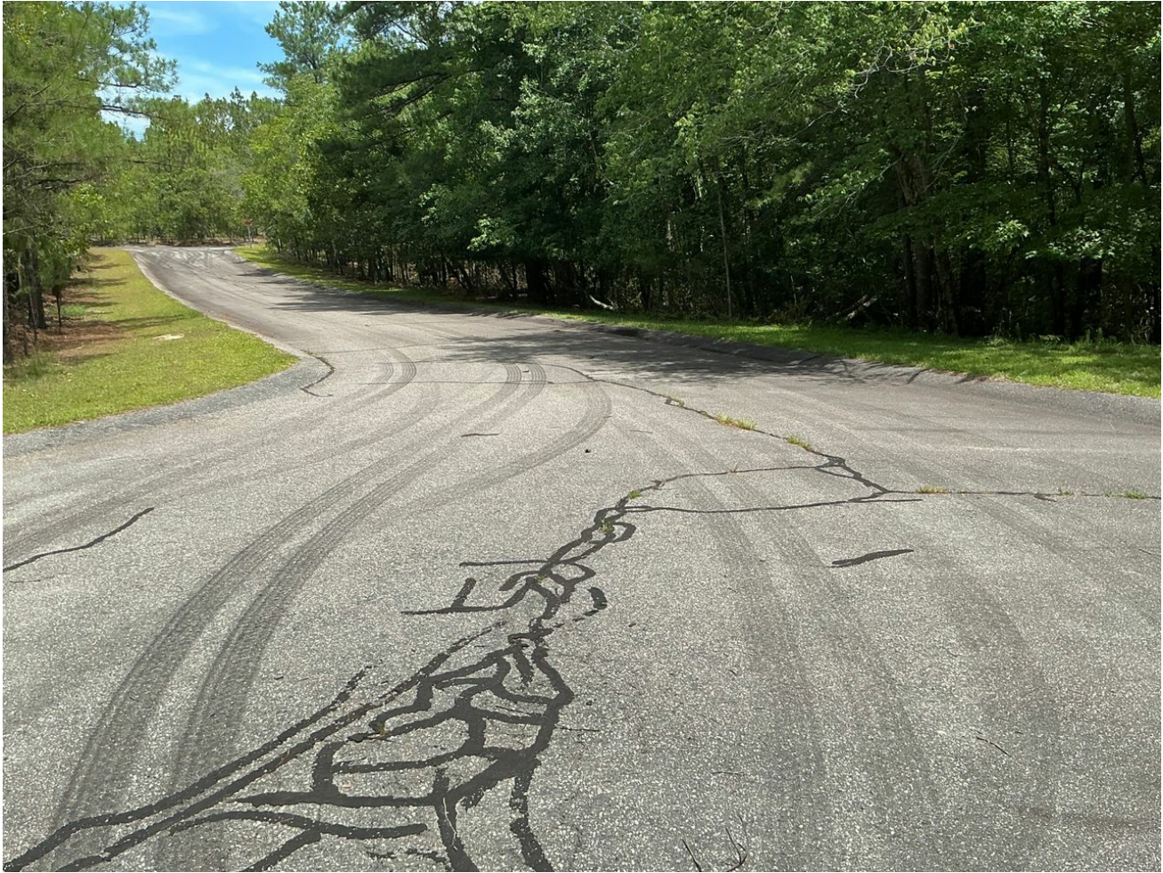
Asphalt Paving & Repairs
