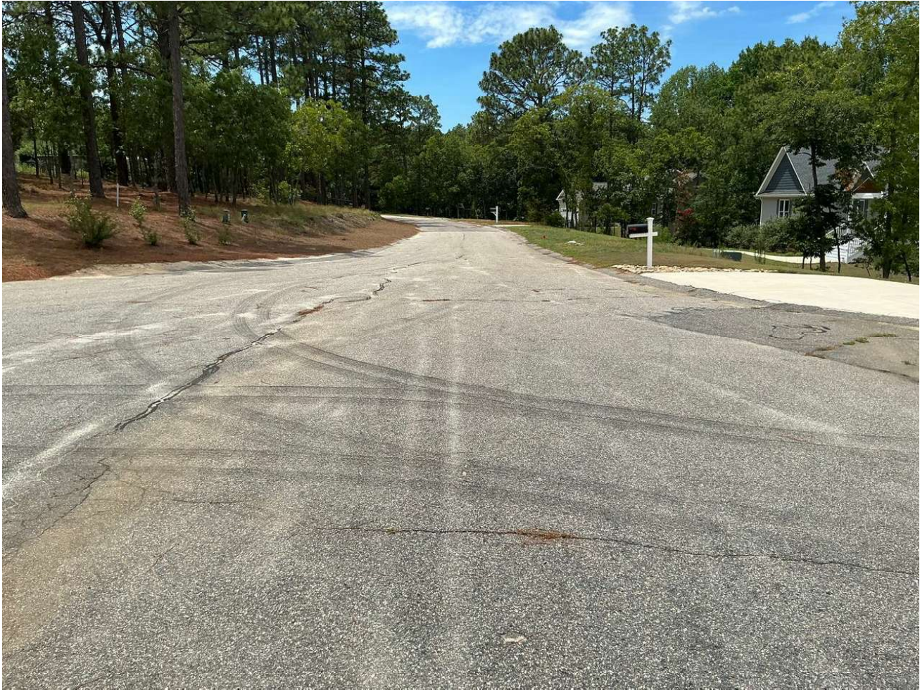
Asphalt Paving & Repairs
