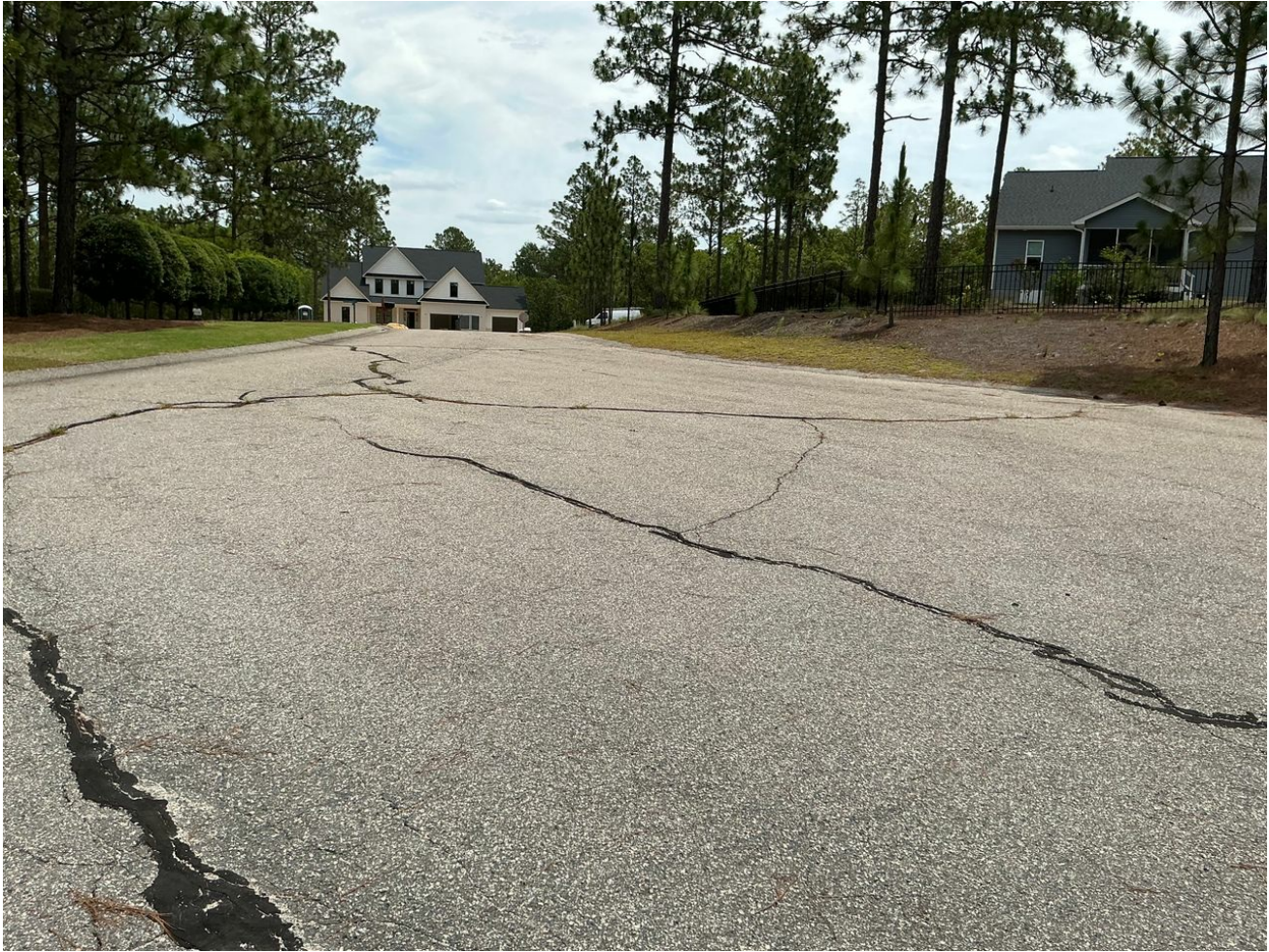
Asphalt Paving & Repairs
