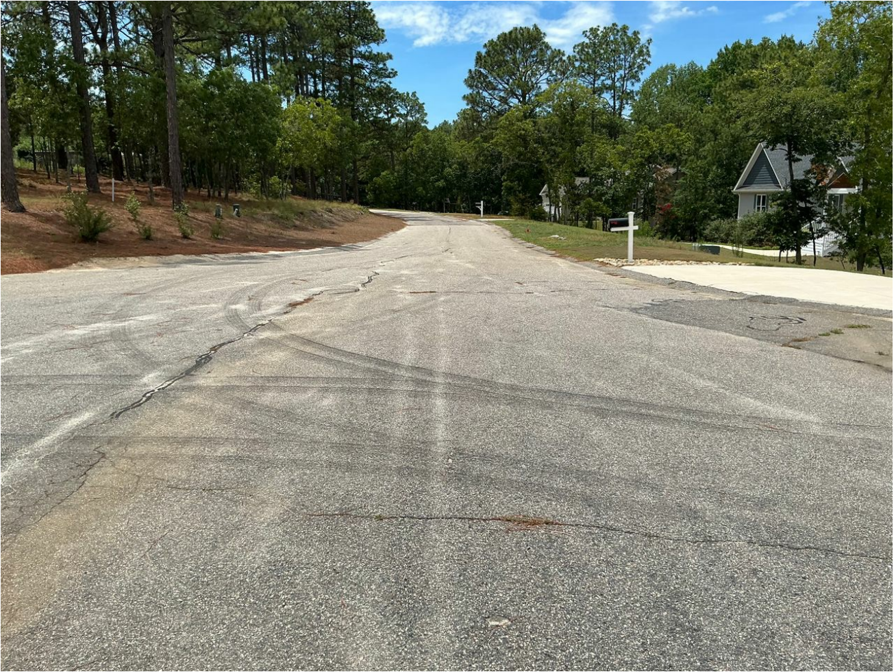
Asphalt Paving & Repairs
