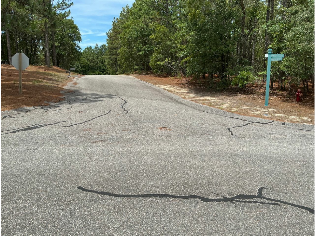
Asphalt Paving & Repairs
